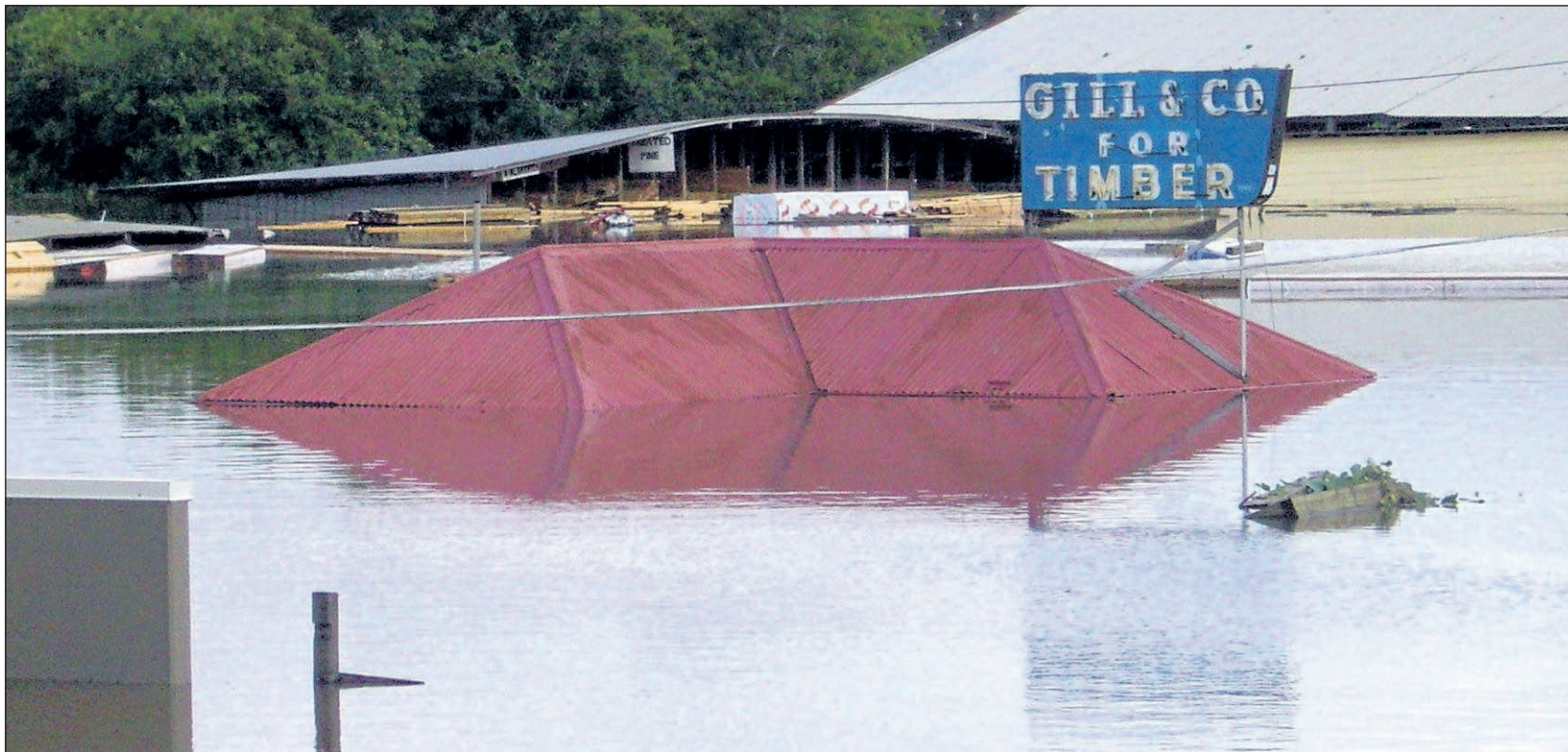
TOUGH TIMES: In 2011 Gill and Co faced a setback with the Brisbane floods. The Rocklea site was completely destroyed and had to be rebuilt.
